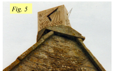
Mounted above the east wall. Here all three faces of the prism are used, facing west, south east and north east. The original dial was in poor condition with the gnomons rusting and delineation all gone (Fig. 4). In 1997 a new dial was mounted, being a near copy of the original with clear delineation and an unusual west gnomon (Fig. 5).
