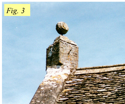
Avening, Glos. (Fig. 3) High on the ridge of the nave at the west end and very badly weathered. The gnomons have gone, as has the delineation. It is so high up that reading it must have been difficult even when new.
