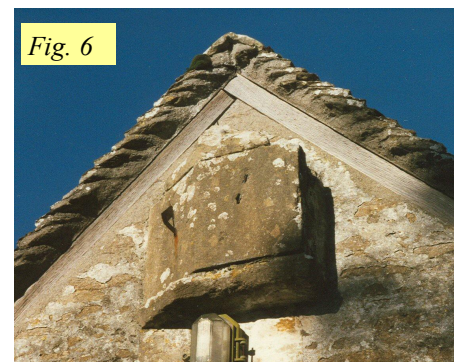
Daglingworth, Glos. (Fig. 6) This church has a Saxon dial, a mass dial and a scientific dial. The scientific one is on the porch and is very early. It is a form of prism dial consisting of two faces declining equally to east and west, the dial then being offset with respect to the wall. The faces are more SSE/SSW and the block has finished up being an untidy shape but just within our definition of ‘prism dial’.
